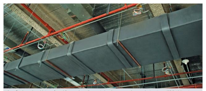
Armaflex has a long history of providing condensation control and energy savings on duct systems. Whilst it is not necessary to have a foil-facing, this added feature can enhance the aesthetic finish and surface durability.
